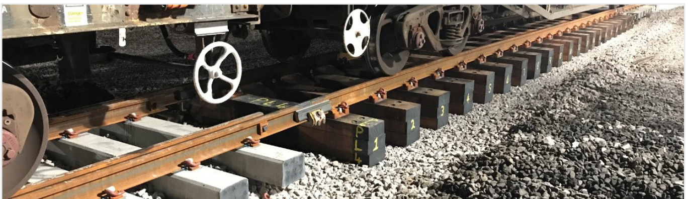
Figure 10: Slave panel design to level rail heights during the installation.
