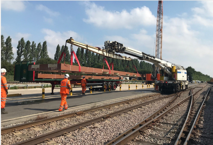
Image 8a: Double bearer sections being lifted onto rail wagons.
