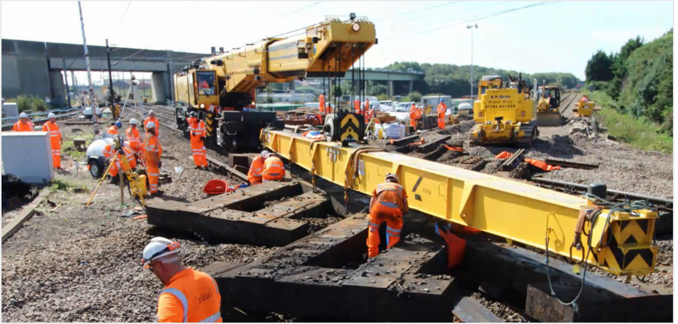
Image 13: One half of the old bearers being removed.
