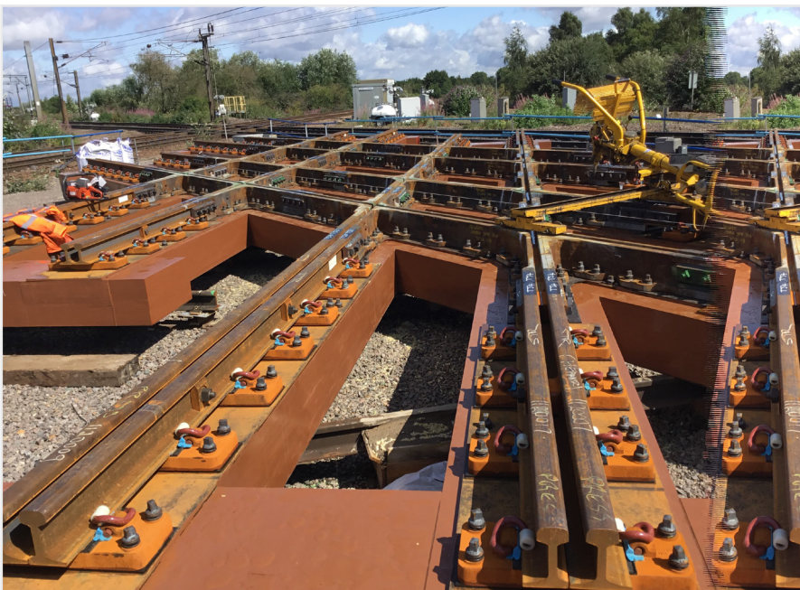
Image 11. Check rail extensions with thickened UCV rail baseplates and Pandrol® e-Plus clips.
