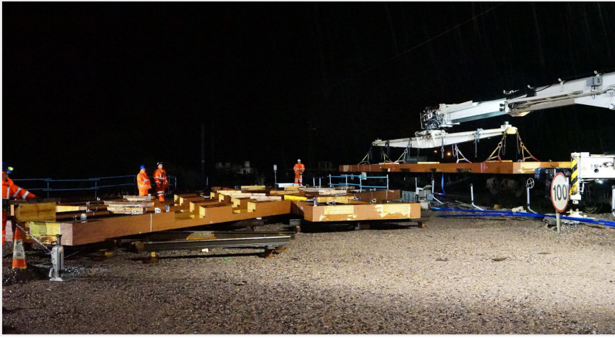
Image 10: Bearer beams being unloaded and re-assembled on site.
