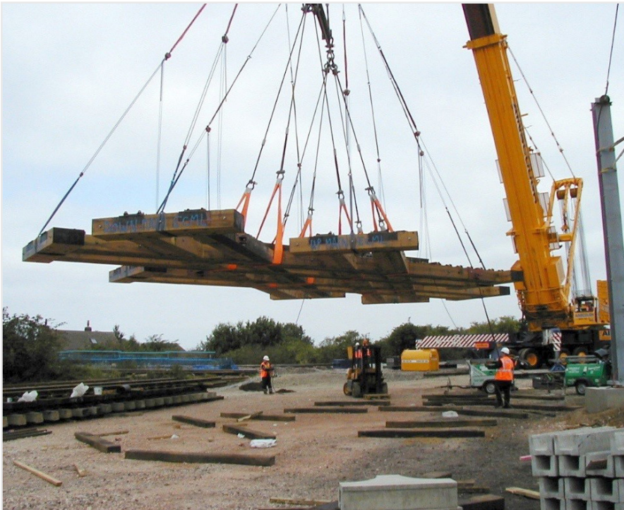
Image 3: The 2003 renewal being installed using a large road crane.
